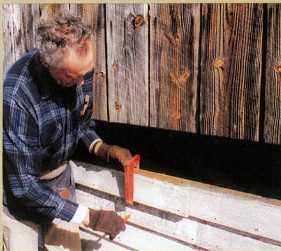
Marking along the buzzard's finger produces more accurate cuts than measuring.
